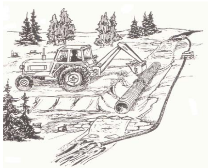
Using a pump-around system to work "in the dry"
