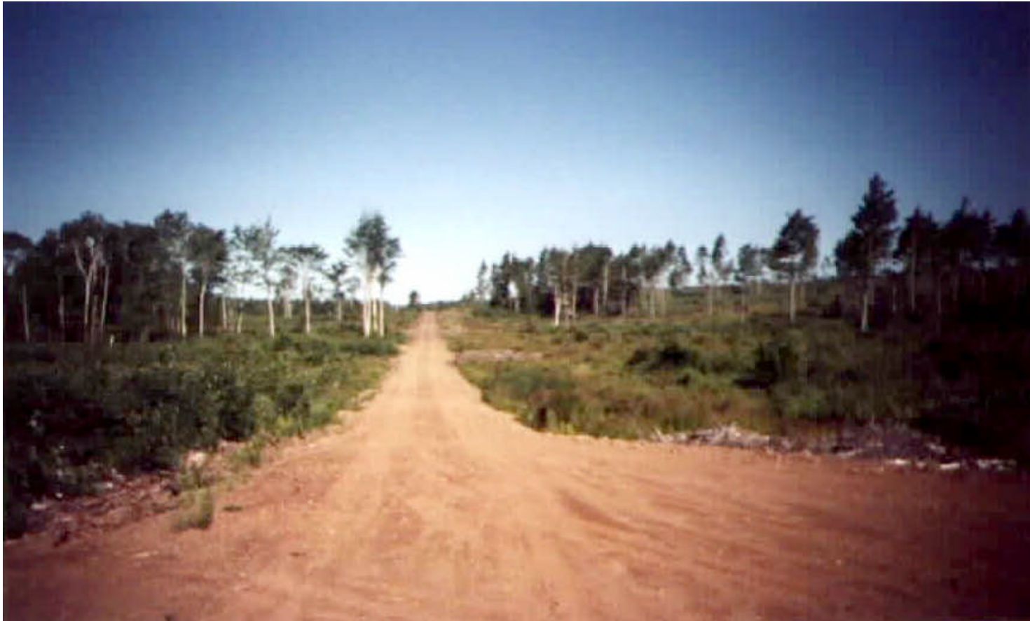
Figure 8. Residual trees may provide soil cover, but do not always prevent soil erosion, especially where forest floor layers are thin. Also, long slopes with silty soil exposed could lead to major soil erosion events along that road.
