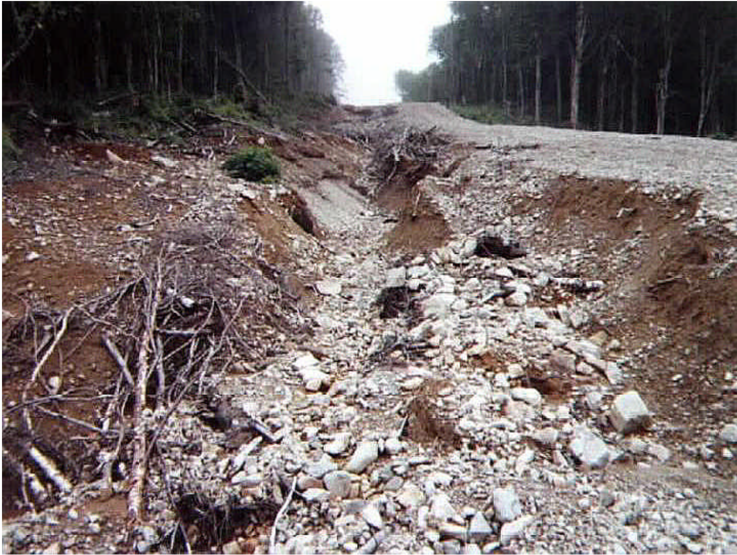
Figure 10. Massive soil movement following haul road failure near Cutblock 10.
